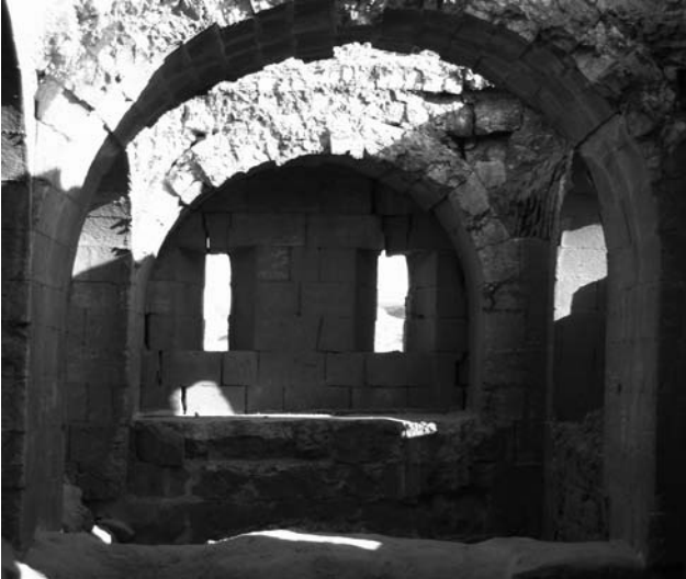
Figure 3 Details inside the gallery.
